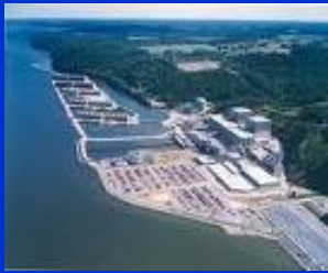
Peach Bottom Atomic Power Station located in southern York County.
